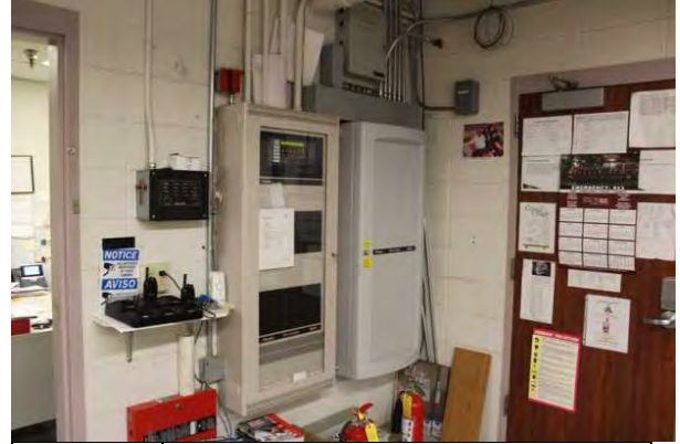
#56 FIRE ALARM CONTROL PANEL, ADDRESSABLE
