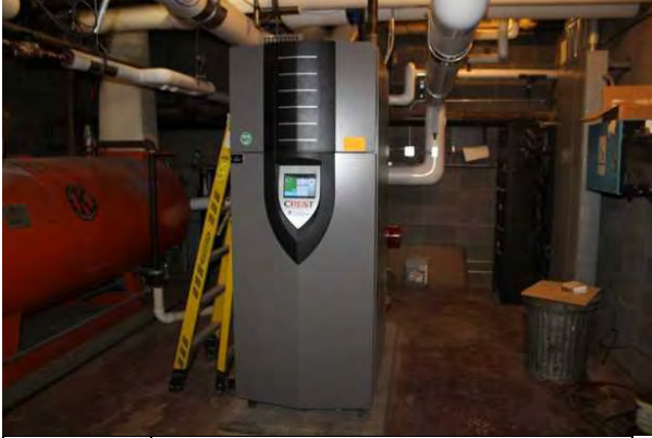
#37 BOILER, GAS, HIGH EFFICIENCY CONDENSING STYLE
