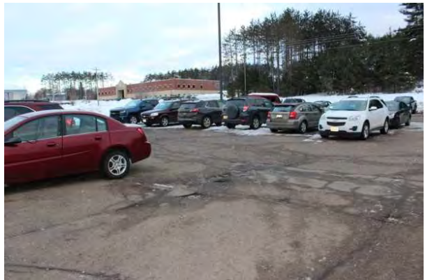
#66 PARKING LOTS, ASPHALT PAVEMENT
