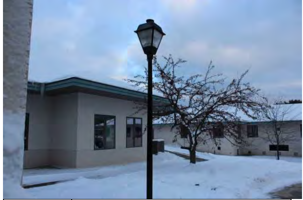
#68 SITE LIGHT POLE BASE
