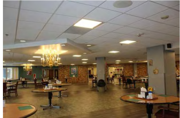
#22 INTERIOR CEILING FINISH, SUSPENDED ACOUSTICAL TILE (ACT)
