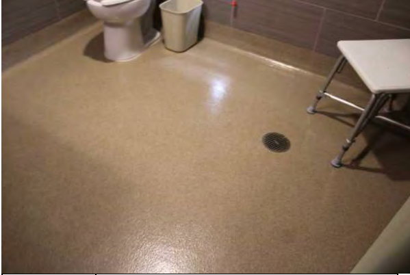
#13 INTERIOR FLOOR FINISH, SURFACE WITH EPOXY COATING
