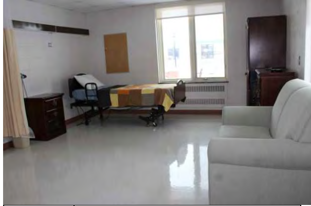
#14 INTERIOR FLOOR FINISH, VINYL TILE (VCT)
