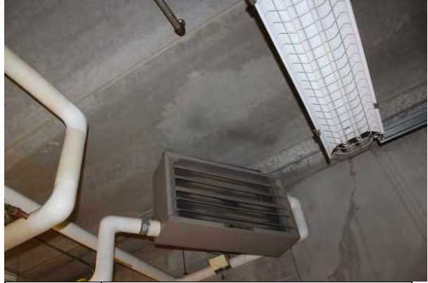
#50 UNIT HEATER, HYDRONIC
