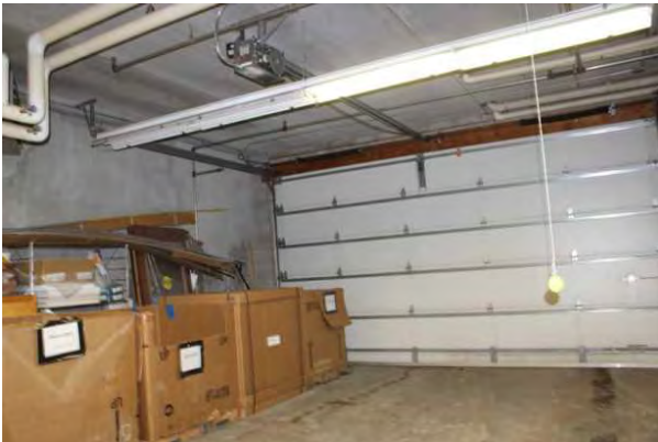
#9 OVERHEAD/DOCK DOOR, ALUMINUM
