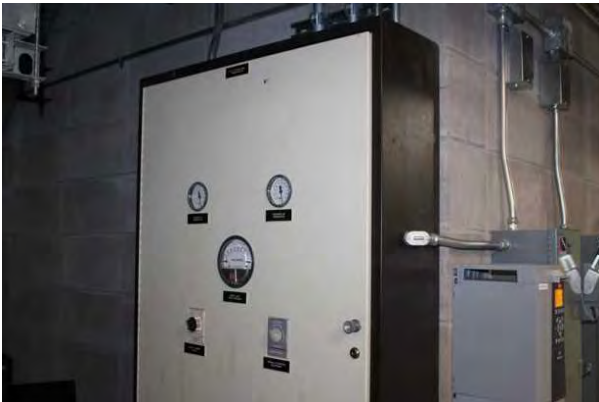
#45 PNEUMATIC CONTROLS
