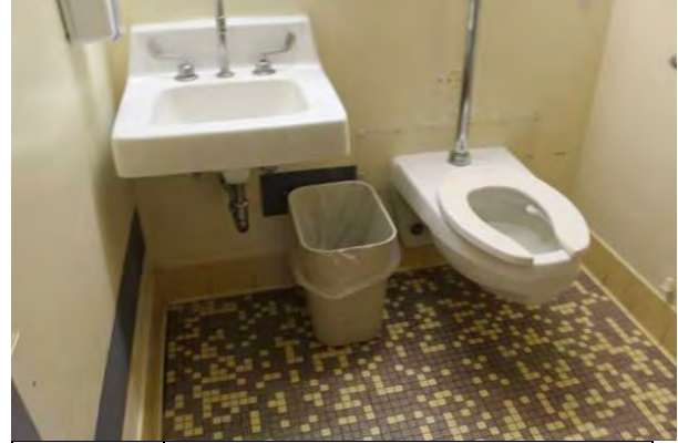
#20 INTERIOR FLOOR FINISH, CERAMIC TILE
