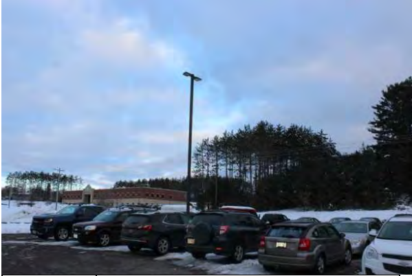
#67 SITE POLE LIGHT, 20' HIGH
