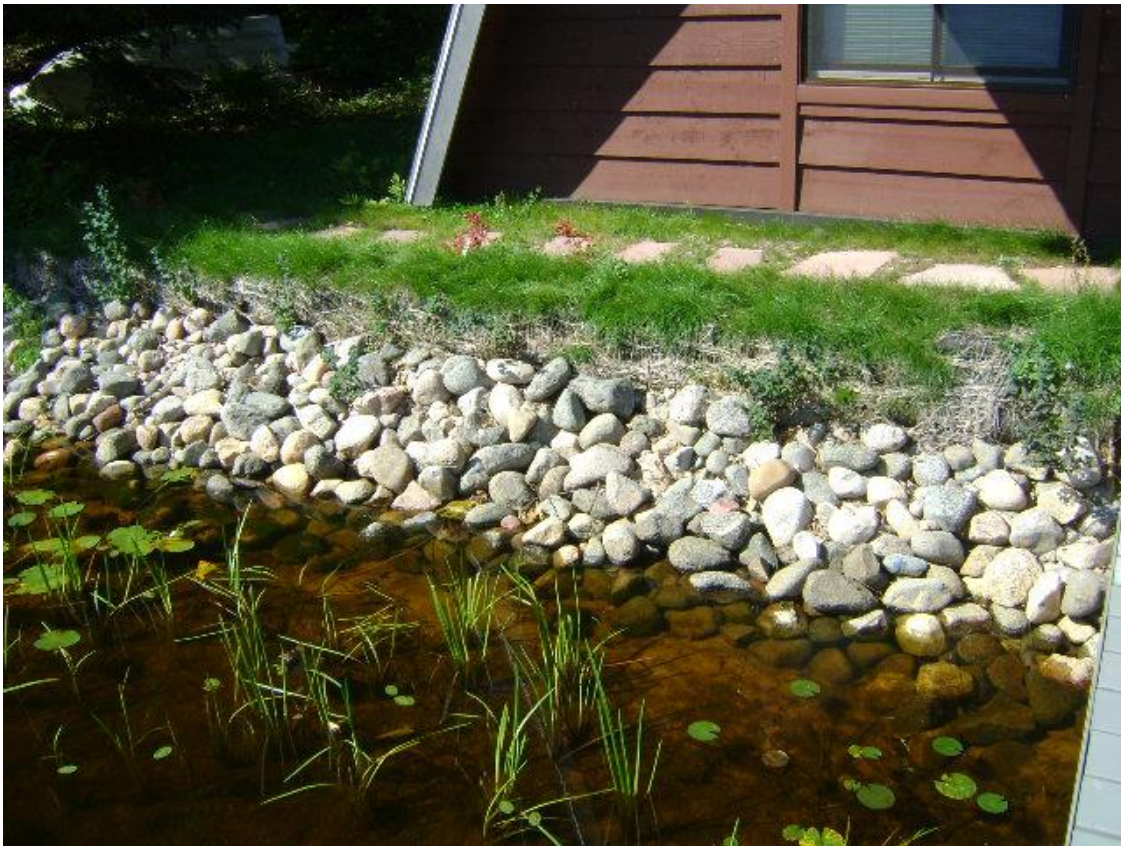
Restored/ stabilized shoreline (County staff photo)
