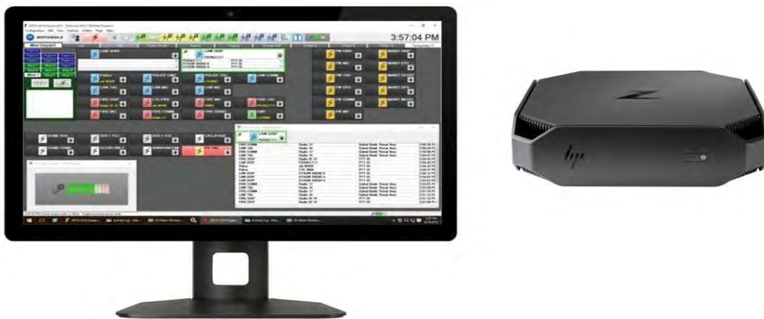
Figure 1-1: MCC 7500E Dispatch Position
