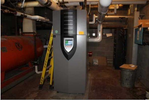
#37 BOILER, GAS, HIGH EFFICIENCY CONDENSING STYLE
