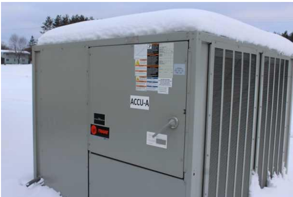
#41 CONDENSING UNIT, SPLIT SYSTEM
