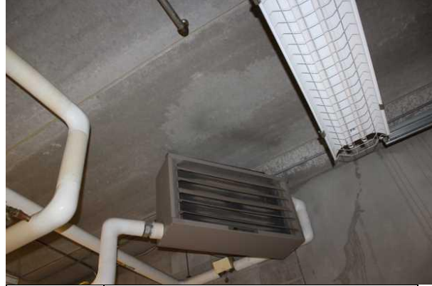
#50 UNIT HEATER, HYDRONIC
