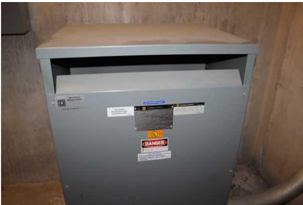
#53 SECONDARY TRANSFORMER
